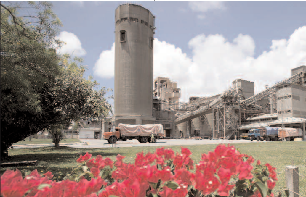
■ Lafarge's plant in Mombasa, where, as part of the company's wider efforts to reduce emissions, 900 hectares of land have been set aside for tree planting
